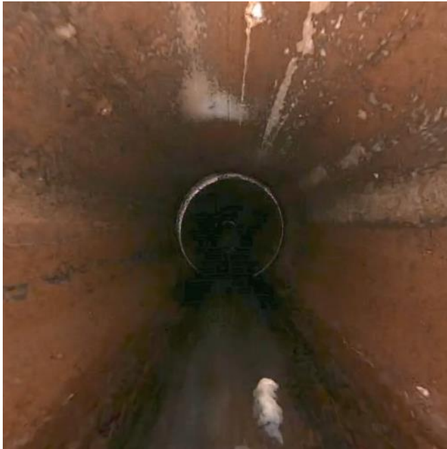
Perspective from inside the pipe
